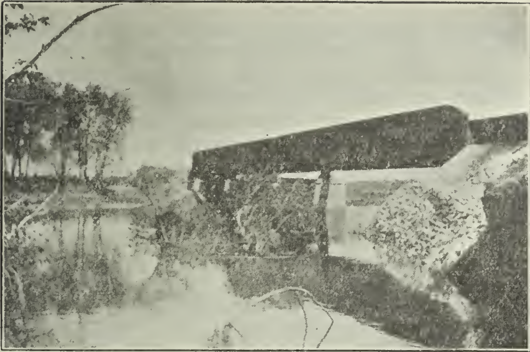
A. Bridge, Looking Down Stream.
